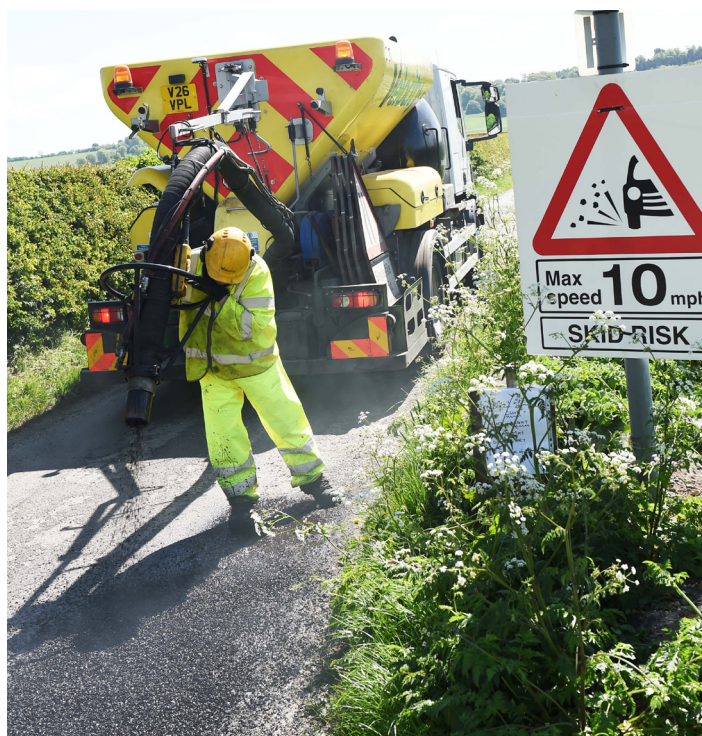
Spray injection machine in use
